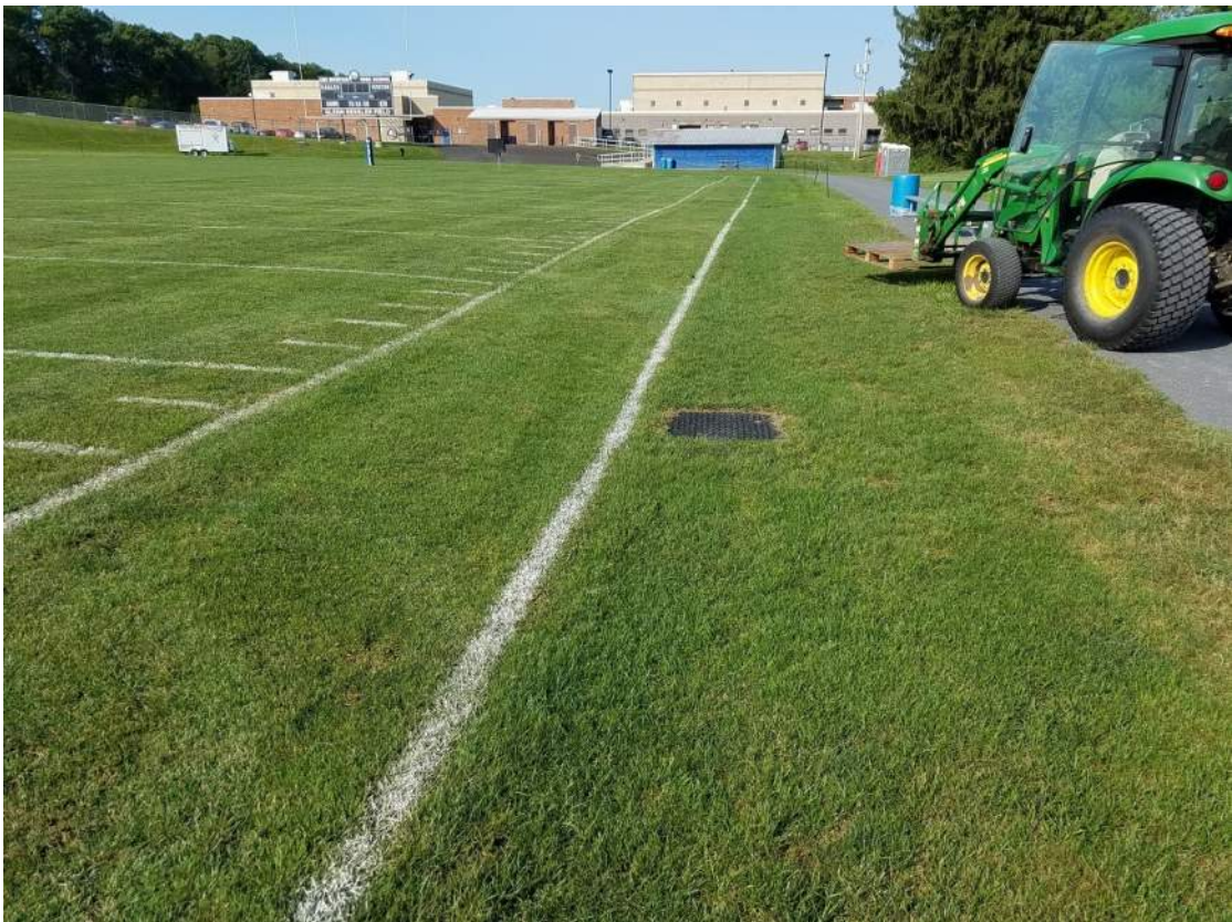
Figure 8: Close proximity of drainage structures to sideline
